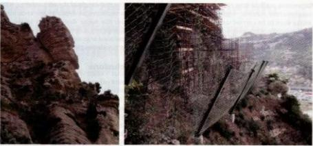
**Fig. 10** Line of catch fences at the base of the conglomerate column providing a barrier to stop rolling or bouncing rocks from reaching the houses at the toe of the slope.
